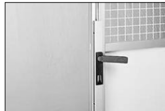
Lock mechanism for double door (p. 10-18)
